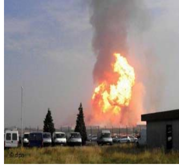
July 30, 2004. High-pressure natural gas pipeline ruptured following recent third party damage: 24 died and 150 hospitalised. Damage to pipeline during the final stages of construction project. ( https://en.wikipedia.org/wiki/Chislenghien )
